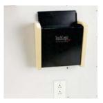
3. Position cabinet and slide onto screws. Tighten screws if required.
