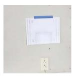
1. Tape template on wall and ensure that it's level.
