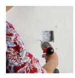
2. Install drywall anchors (4) and screws (4). Tighten screws within 1/16" of anchor.
